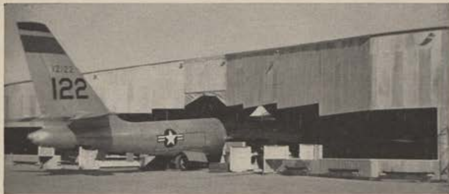
Portable steel maintenance dock for B-47s built by Luria Engineering Company.
