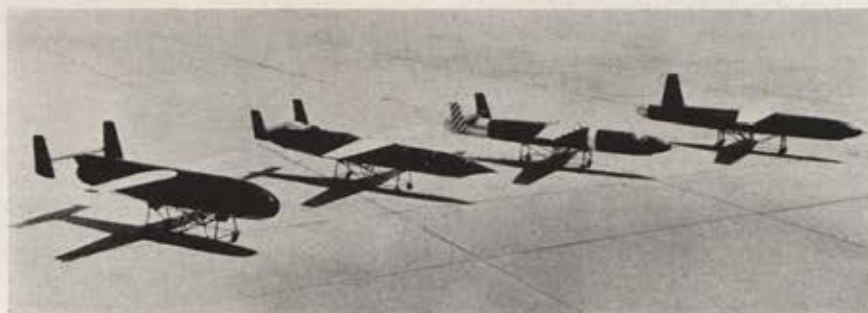
From left: the YQ-1B jet drone and its predecessors—XQ-1A; XQ-1 (Modified); and the XQ-1. They are products of Radioplane Co., a subsidiary of Northrop.
