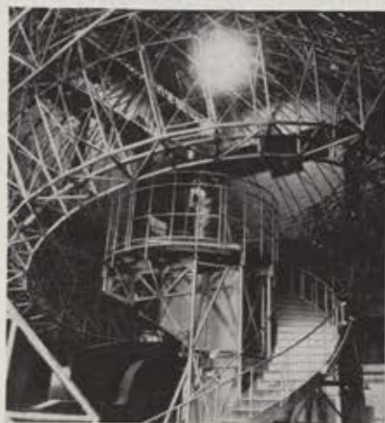
Interior of the Link High-Speed Navigation Trainer, looking up toward the "stars" of the northern hemisphere.
