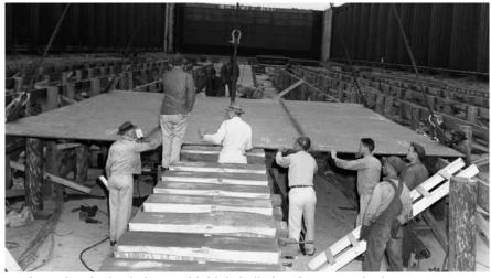
Workmen lay the keel plate and initial shell plate for USS *United States* at Newport News Va., in 1949. The carrier was canceled days later.
