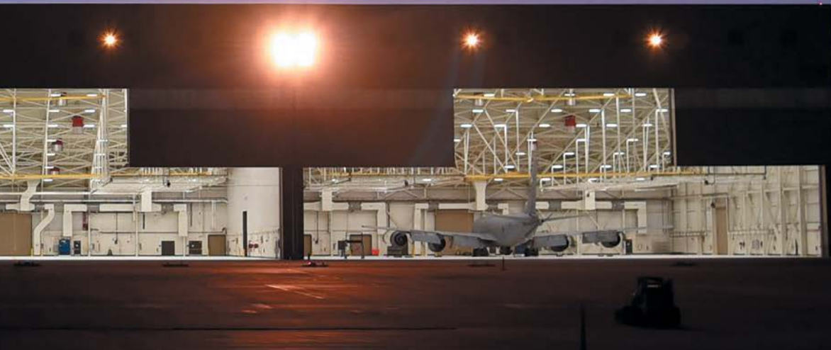
McConnell AFB, Kan., boasts this three-aircraft hangar for KC-46s.
