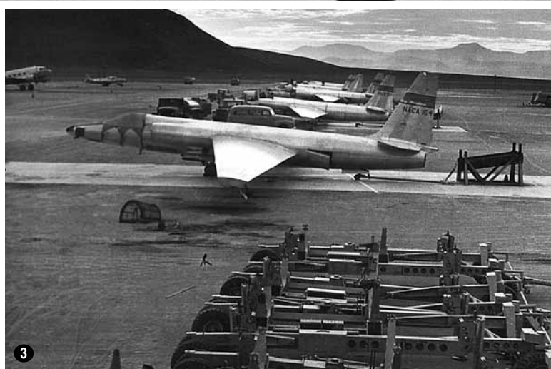
111 A U-2 receives a postmission check. The aircraft's wings were patterned after those on gliders, to obtain maximum lift. Early test flights were confined to an area within 200 miles of Groom Lake; a pilot whose single engine flamed out could make a dead-stick landing back at the secret base. 121 Behind the fiberglass panels on the nose of this early U-2 were sensors that collected signals intelligence on Soviet radars tracking the airplane. These data were collected and analyzed after each mission, to plot future routes away from defenses. 131 A half-dozen U-2s wore NACA markings early in flight test. 141 U-2s were built by Lockheed at Burbank and Palmdale, Calif., then loaded in C-124 Globemaster IIs and reassembled at Groom Lake for test and operations.
