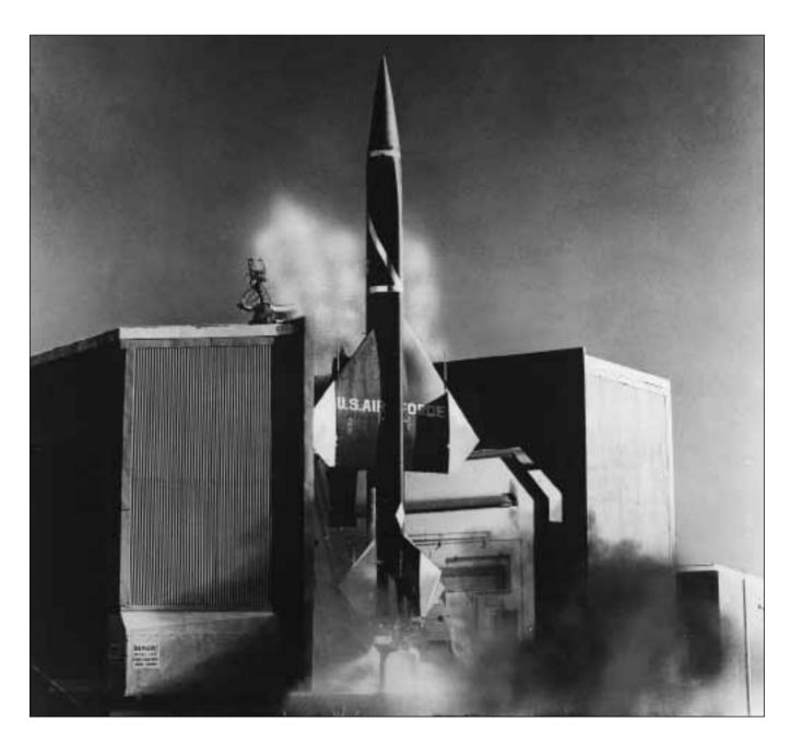
In the 1950s, the Soviet bomber threat produced calls for a stronger North American air defense. USAF responded, in part, with BOMARC, the world's first long-range, supersonic, anti-aircraft missile. The pilotless BOMARC ("BO" from Boeing, "MARC" from the Michigan Aeronautical Research Center) was designated XF-99, then IM-99, and then CIM-10A. The system be-
