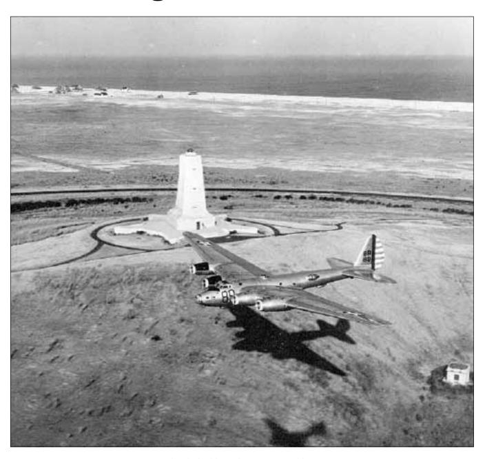
At Kitty Hawk, N.C., an XB-15 makes a low pass—sometimes called "cutting the grass"—near the monument to the 1903 Wright brothers' flight. The Boeing aircraft was a one-of-a-kind and first flew in October 1937. Its innovative features included a sleeping area for the crew and a flight engineer's station, as well as enough room in the wings for the aircrew to access the engines in flight. The XB-15 could carry a
