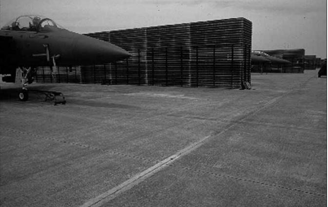
Kwangju has only a few permanent aircraft shelters available. Above, protective steel revetments not only provide some protection for the 90th's F-15Es but also create a more secure environment for maintenance crews as they work on the aircraft.
