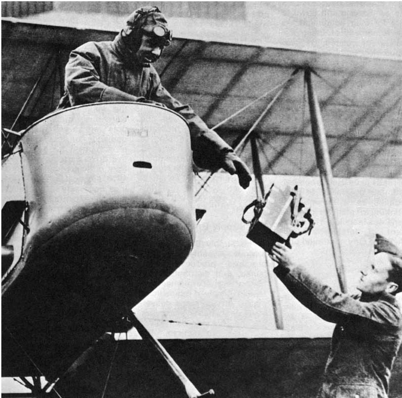
When America entered World War I, military aerial photography virtually was unknown, but it emerged as a major weapon. The Army Air Service in 1917 created a Photographic Section, and pilots flew regular photo sorties. A camera was mounted in the fuselage and was operated by a photographer called an air ob-
