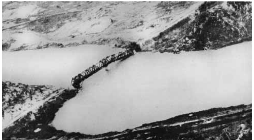
The Thanh Hoa Bridge’s western end was knocked into the Song Ma in April 1972. In May, 2,000-pound and 3,000-pound laser guided bombs blasted it off an abutment.
