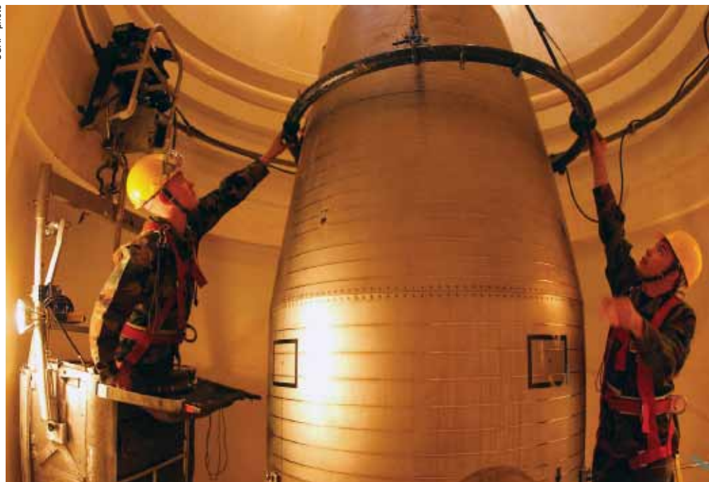
Missile maintenance technicians work on a Minuteman III ICBM in its launch silo during a nuclear surety inspection at Malmstrom AFB, Mont.
