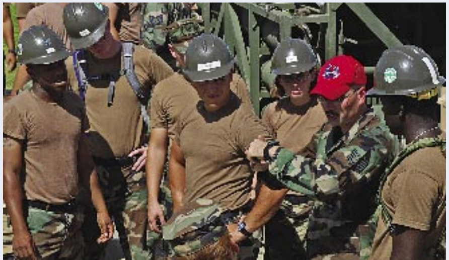
USAF RED HORSE airmen and Navy Seabees in a joint training exercise at Kadena AB, Japan, in September. More than 87 Seabees participated in the rapid runway repair exercise and trained with Kadena's RED HORSE engineers on a variety of tasks, from repairing craters to foreign object removal and ordnance detonation.
