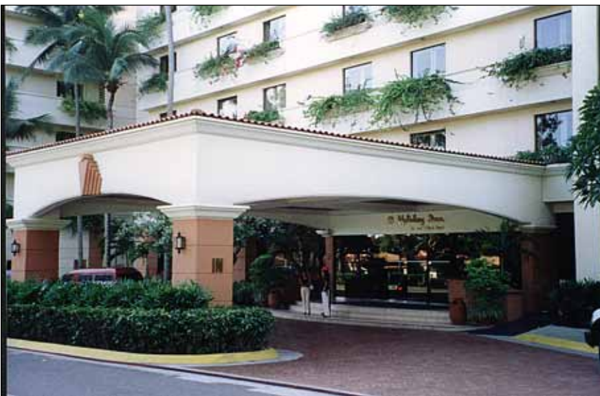
After USAF closed down Clark, it became a special economic zone that attracted Asian investors. The base’s transformation included a makeover for Chambers Hall, once the bachelor officers’ quarters, now a five-star Holiday Inn.
