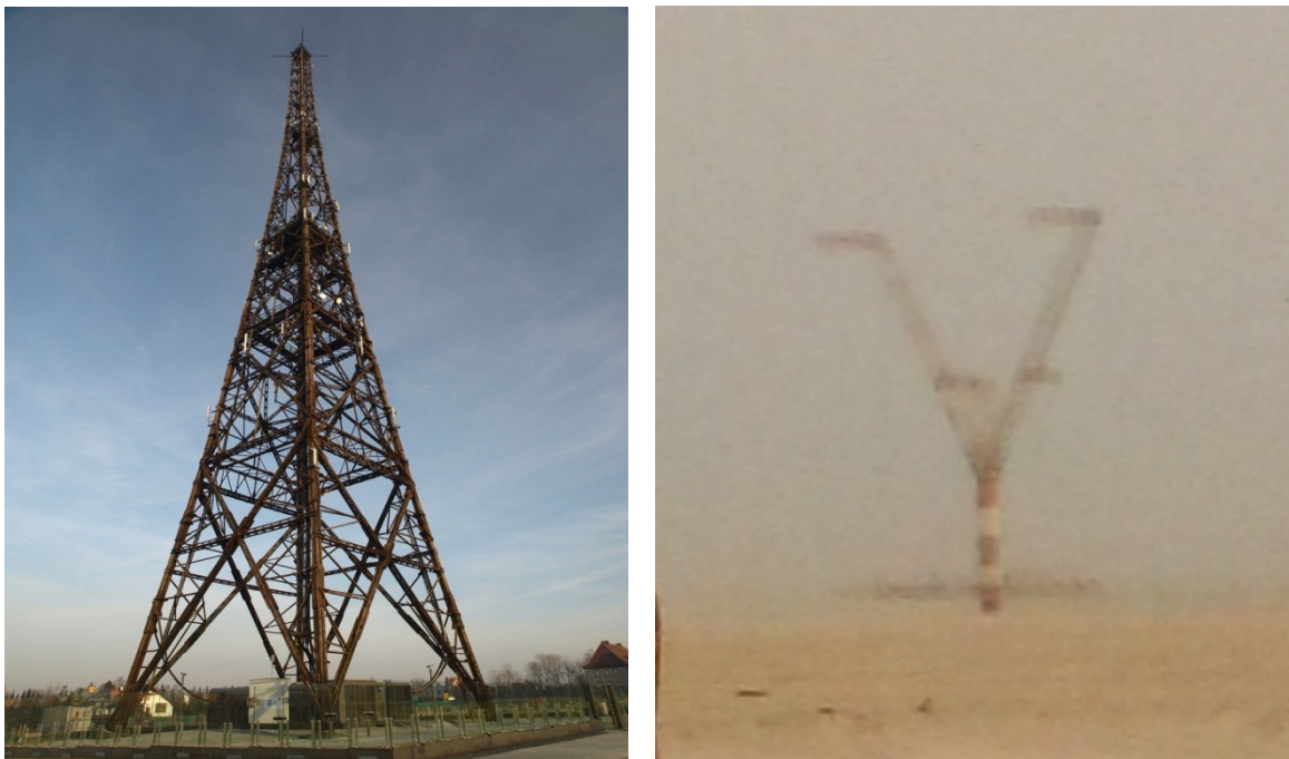
Figure 11. The left image shows a “typical” tower, wide at the bottom and narrow at the top. The right image shows the “Y” tower located north of the tower array.
