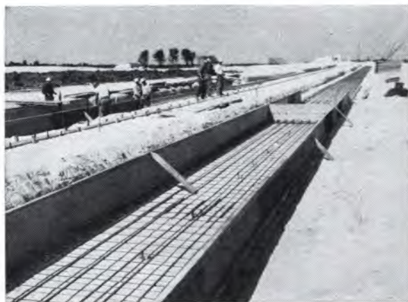
Concurrency concept in site construction is demonstrated in this view at Cape Kennedy, Fla., where workmen are preparing railbeds leading from Titan III booster assembly area to launch pad, while the components of Titan III are still under development.
