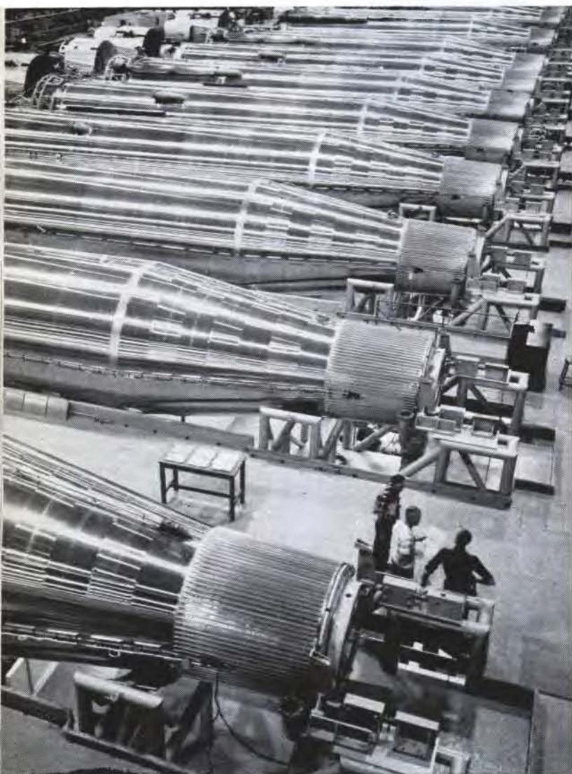
Atlas production line at San Diego plant. Missiles were nested in elevated docks. At upper left, booster sections have been pulled back to install rocket engines. By December 1955, fifty-six major contractors were engaged in the Atlas program alone.
