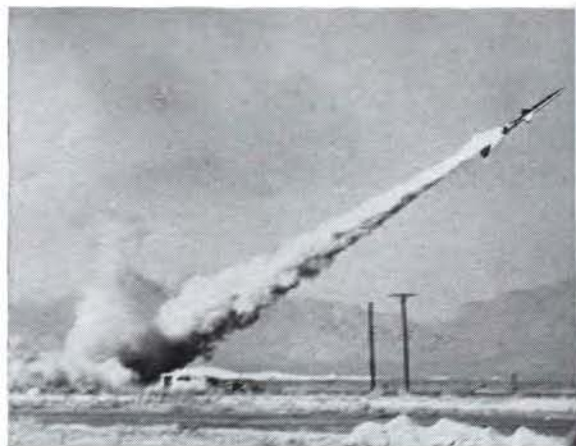
A GAPA firing at Alamogordo, N. M., in 1953. Photo shows angled takeoff of supersonic research vehicle, capable of reaching speeds of 1,500 mph. But the GAPA was never placed into production.
