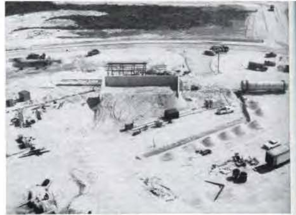
Unlike Atlas sites, each of which stores its own missile fuel, groups of three Titan I launchers are served by a central tank, while portable tankers fuel Titan IIs. Here construction begins on the still more advanced fuel storage system for the new Titan III.
