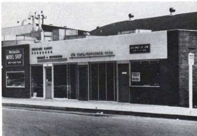
This little storefront at Westchester, Calif., represented the corporate beginnings of the Ramo-Wooldridge Corp. in the early 1950s. The new company's technical staff, serving as advisers to General Schriever's Western Development Division, coordinated efforts of several large companies.
