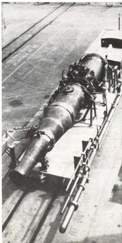
The Tory II-C reactor, measuring 4.7 feet in diameter and 8.5 feet in length is in the test ducting at right. It is a complete flight weight unit which produced 600 megawatts of power last May for five minutes under simulated Mach 3, sea-level flight.
