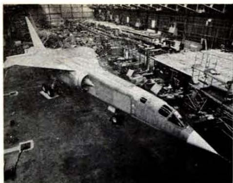
The TSR-2 is scheduled for rollout early this year. Its highly sophisticated electronic systems will enable it to hug the ground at high speed and in total darkness.
