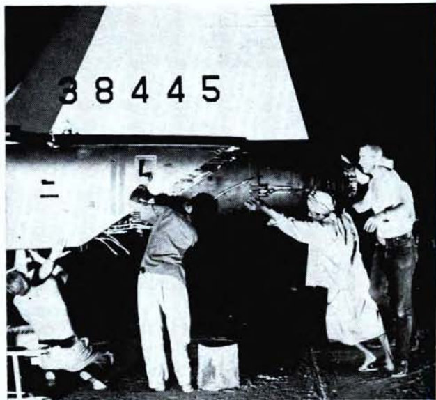
Emergency engine change in Saudi Arabia during recent F-5 demonstration tour illustrates the relative ease of F-5 maintenance. Each engine weighs less than 600 pounds. Changes have been made in the field by four-man crews without use of special tools or without even crude hoists.
